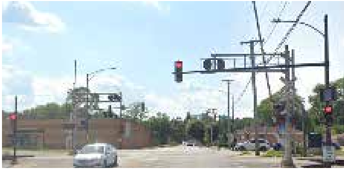
This is a photo of 107th Street in Chicago on the Rock Island
